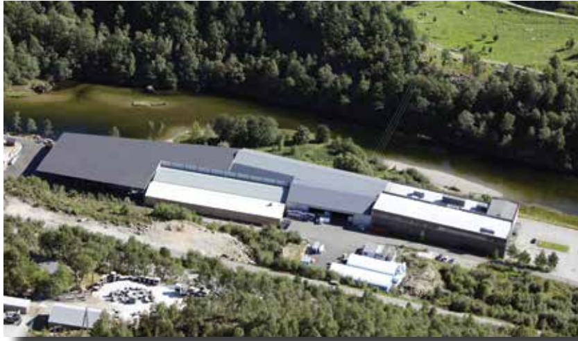
Factory in Bjerkreim, Norway. Total of 10.000 m 2 manufacturing area.
